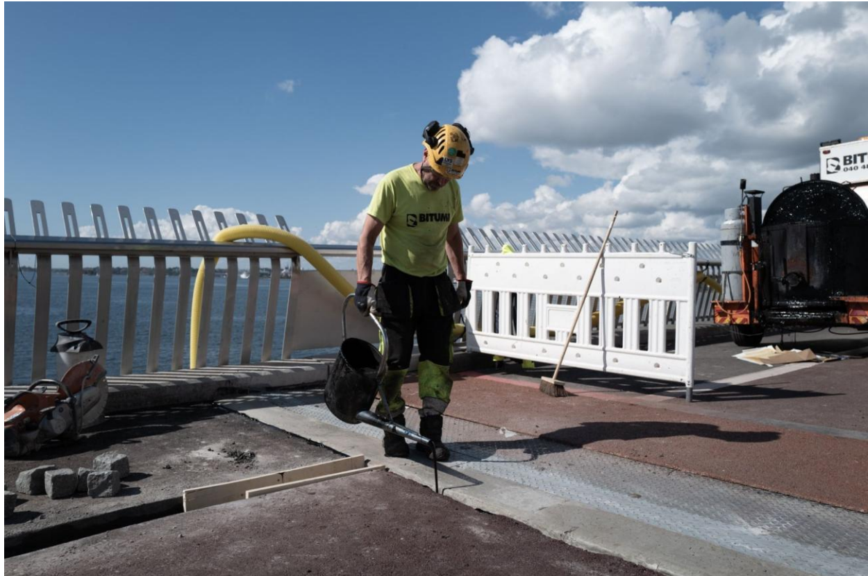
Putting finishing touches on the thermal expansion joints (photo courtesy Nilas Meltio / HS)
