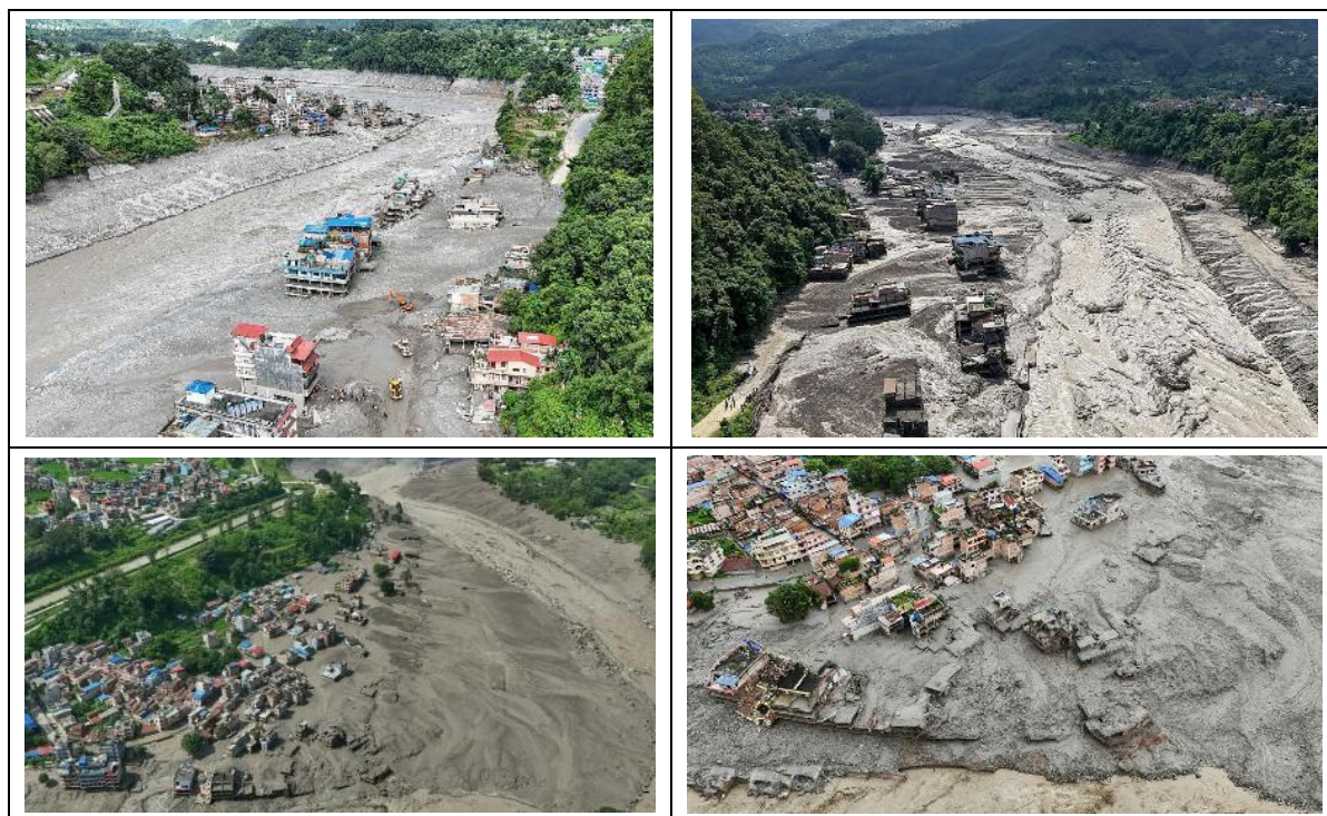
Figure 2: Flood and debris impact along the Trishuli corridor following the 26 August 2026 event. The concentration of settlements and infrastructure along the river corridor illustrates the narrow spatial and temporal margin available for protective action.
