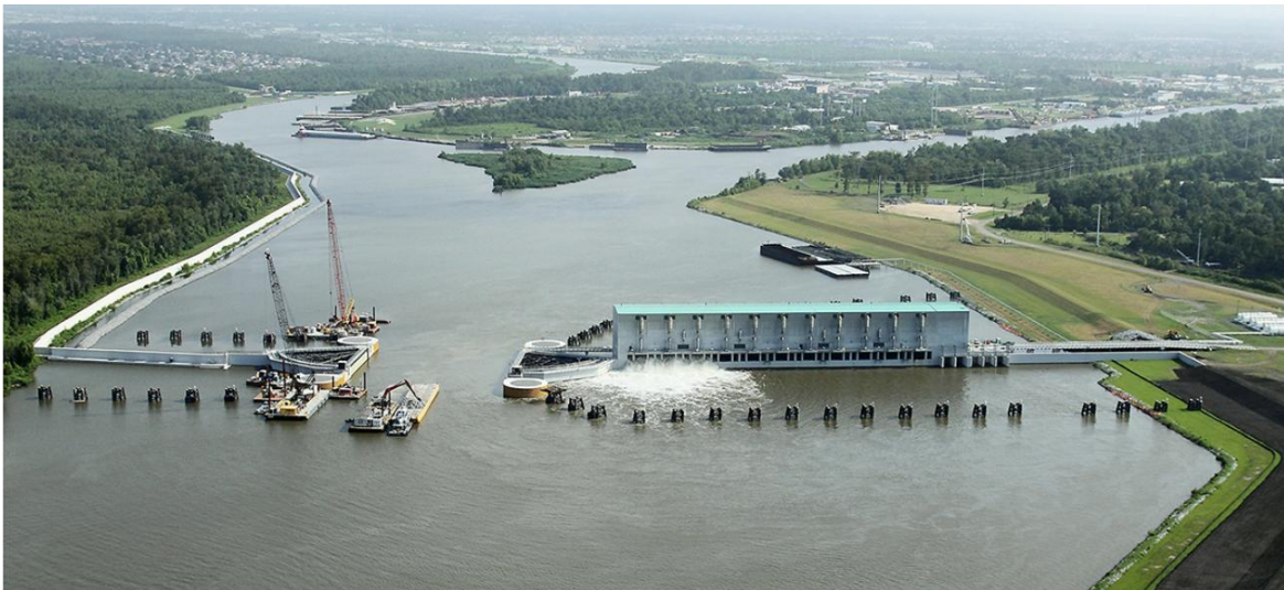
Figure 6. This image shows the West Closure Complex. These structures prevent high water entering the Harvey and Algiers Canals from the Gulf on the west side of New Orleans. It includes the world's largest drainage pump station and the nation's largest gated structure spanning 225 feet with two 700-ton sector gates. (Source: U S Army Corps of Engineers)
