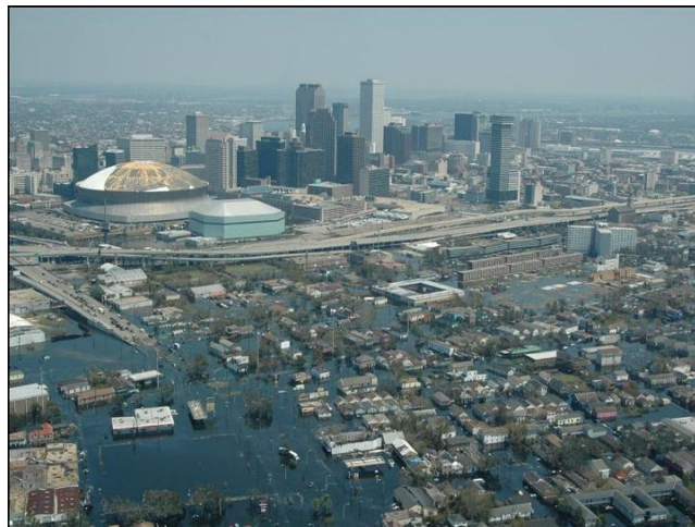
Figure 2. Katrina flooded approximately 80% of New Orleans and damaged 34 of the 73 pumping stations that drain water from the city. New Orleans suffered 1800 fatalities and up to $200 B in total economic losses. (Source: Corps of Engineers)
