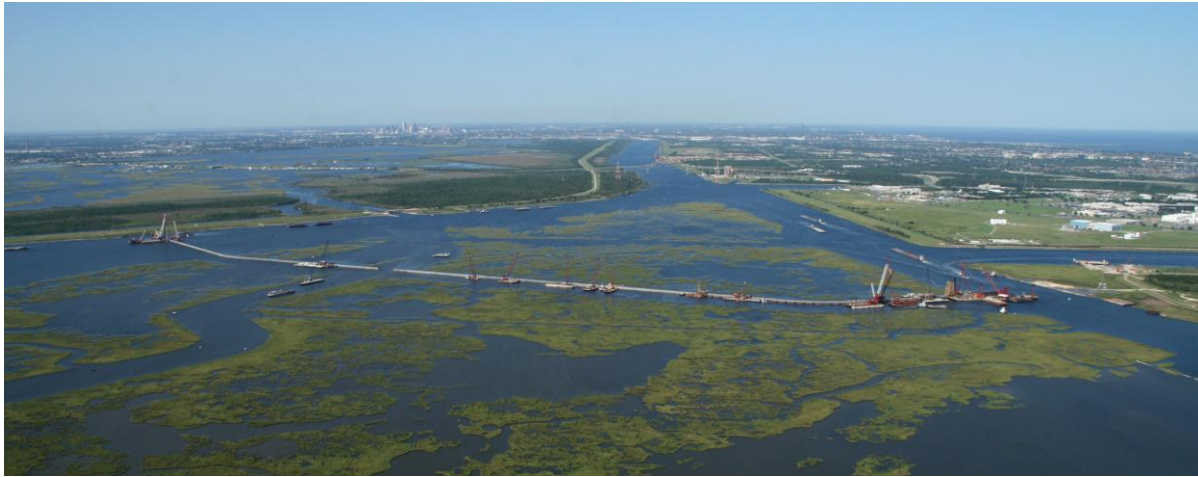
Figure 5. The Inner Harbor Navigation Canal Surge Barrier at Lake Borgne was one of the largest in the world and was executed using the largest Design-Build contract in the Corps' history. Total cost exceeded $1B. This structure has a foundation 60 feet deep and rises over 26 feet above normal water levels. (Source: U. S. Army Corps of Engineers)
