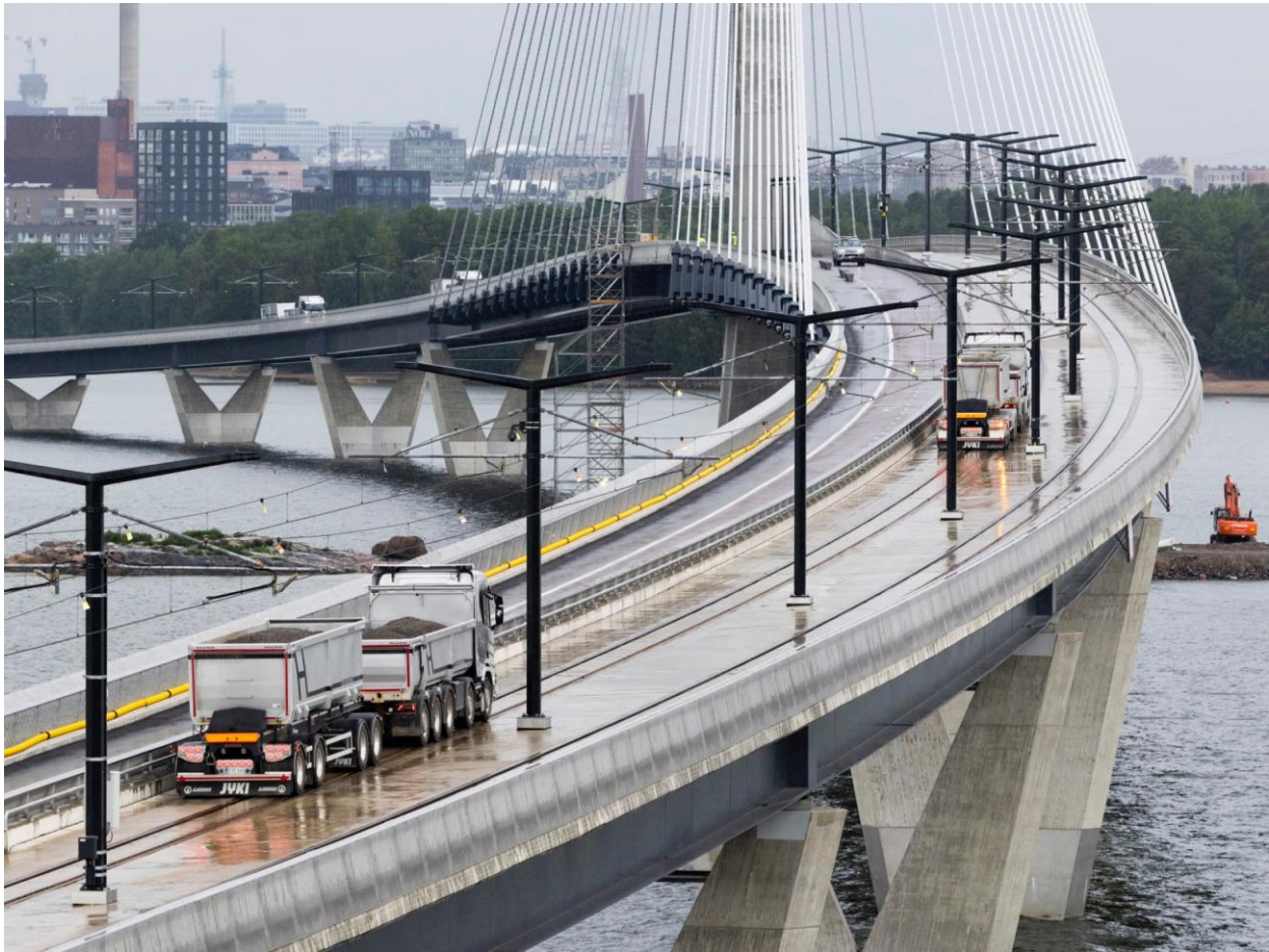
Load testing of Kruunuvuorensilta bridge (photo courtesy Rio Gandara / HS)
