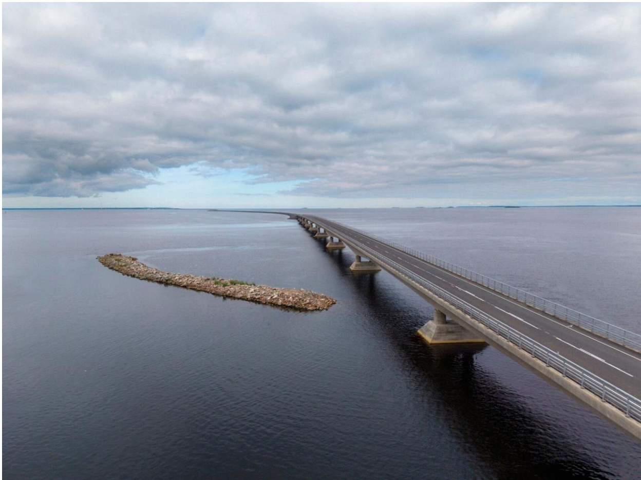
Hailuoto causeway bridge is now open for traffic (photo courtesy Antti J. Leinonen)
