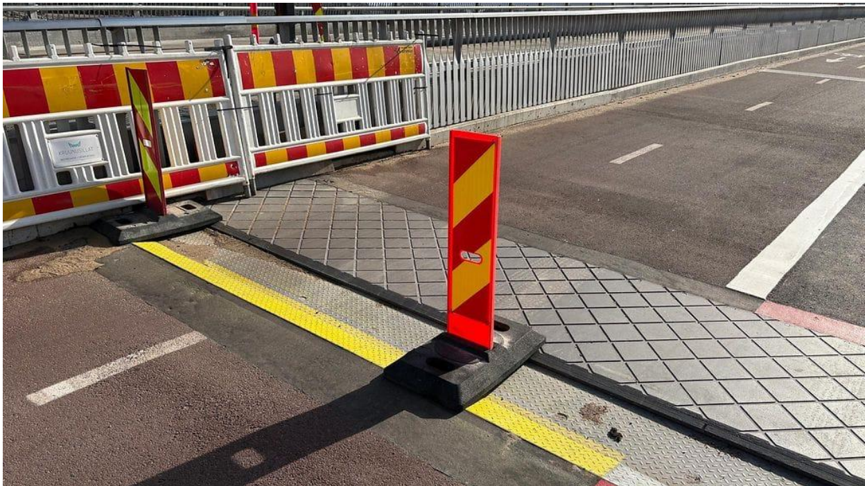
Kruunuvuorensilta bridge thermal expansion joint (photo courtesy Sara Güven / MTV)
