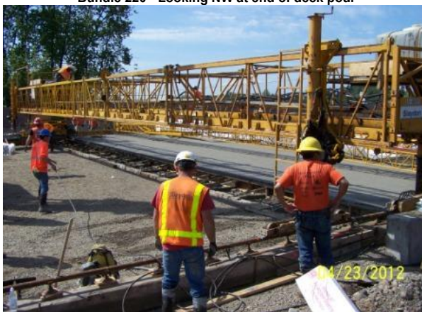
Bundle 220 - Looking NW at end of deck pour
