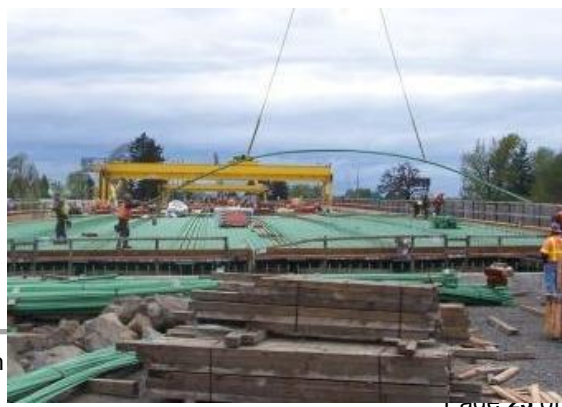
Bundle 210: Installing epoxy coated rebar
