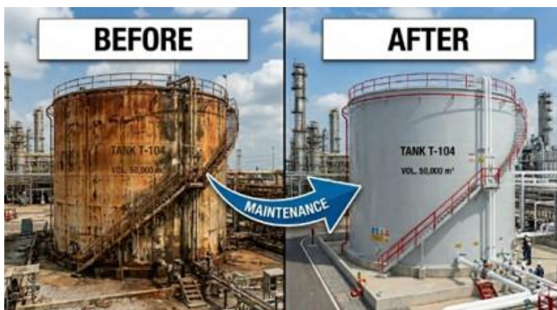
Figure 4. Oil Tank Before and After Maintenance 11
