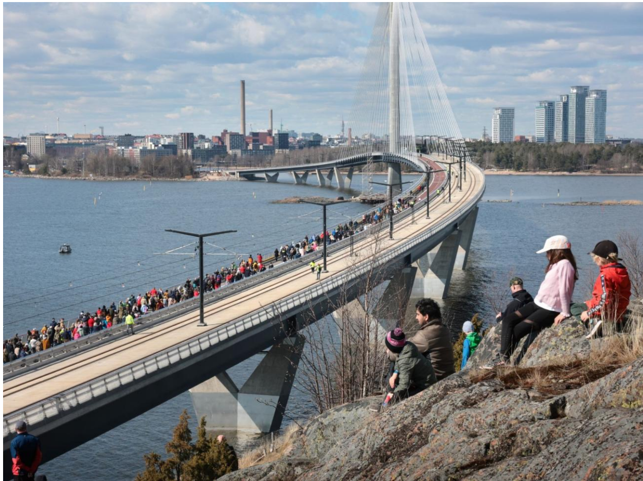
Kruunuvuorensilta bridge was opened for pedestrian and bicycle traffic on 18 th April 2026 (photo courtesy Kimmo Taskinen / HS)
