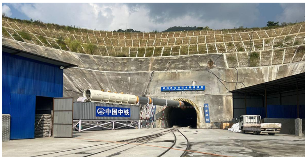
Sunkoshi-Marin Diversion 13.3 km tunnel breakthrough was completed in May 2024
