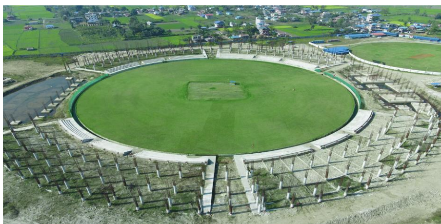
The international cricket stadium is under construction since 2018
