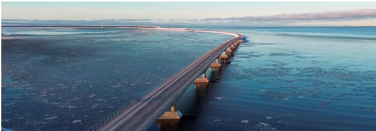
Hailuoto causeway bridge in spring (photo courtesy www.vayla.fi )
