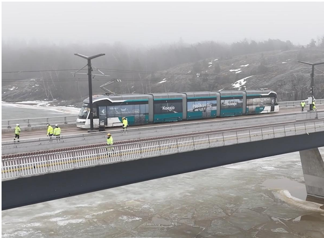
First tram crossing the Kruunuvuorensilta bridge on 17 th March 2026 (screen capture of a video by Sami Kero)
