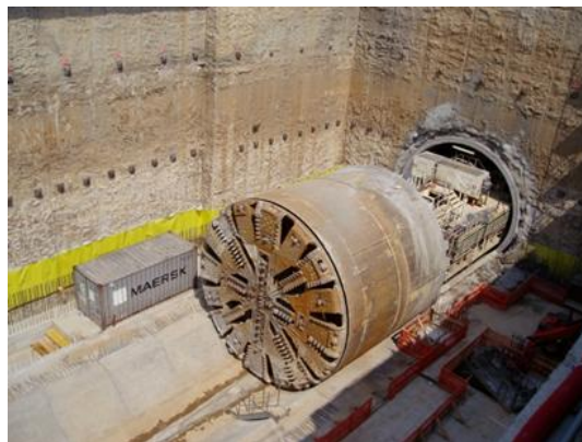
Figura 2 TBM operations
