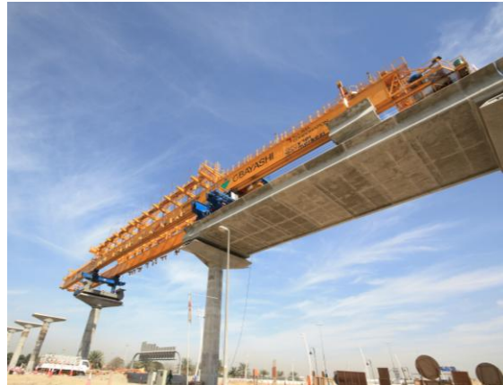
Figura 3 Deck erections
